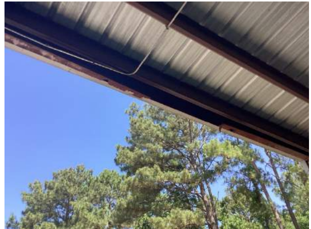
Rust at gutter interface
