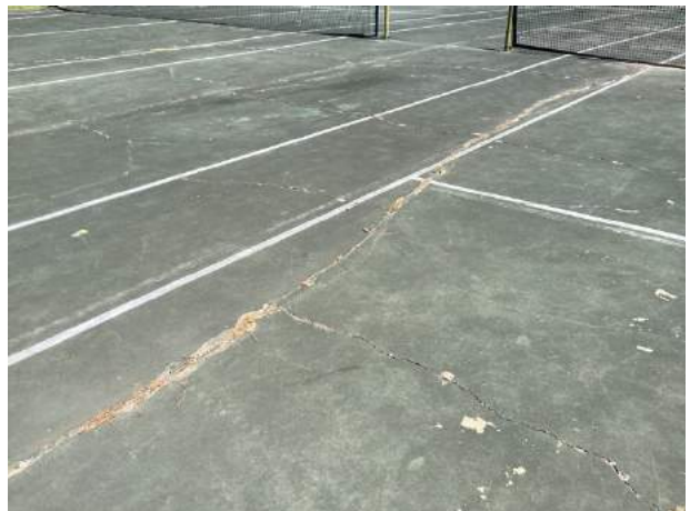
Court trip hazards and cracks
