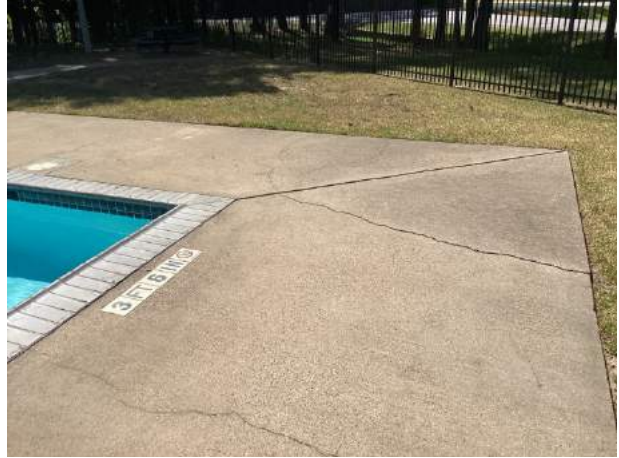
Concrete cracks
