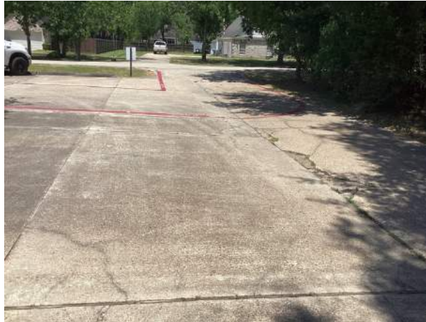
Cracks and settlement at office parking area
