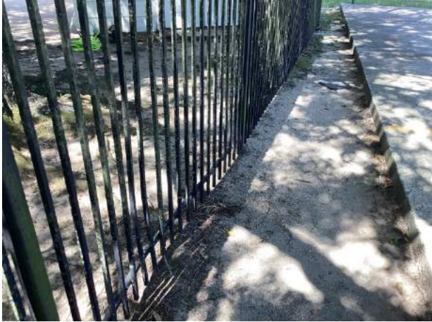
Fence picket damage
