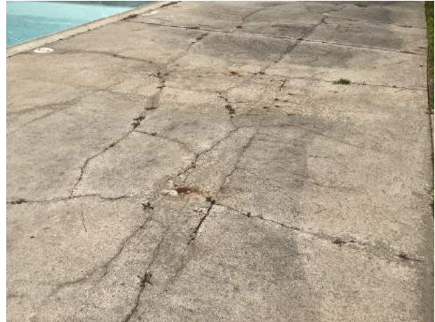
Excessive cracks at the Nickaburr Creek pool
