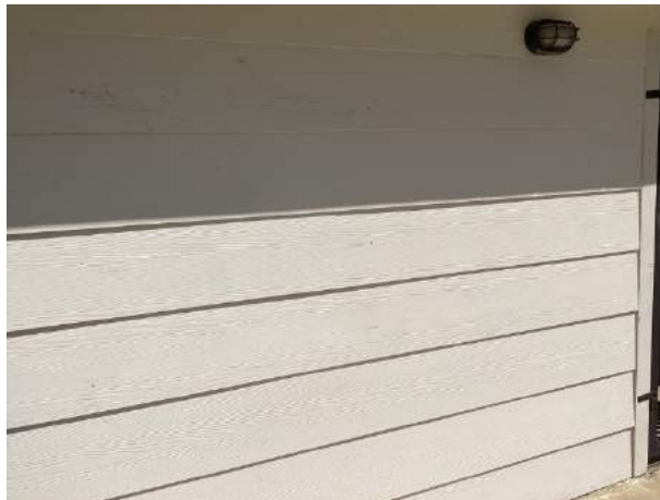
Fiber cement siding overview
