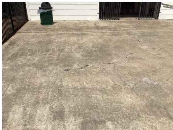
Concrete cracks
